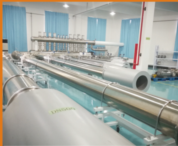
Diameter DN500 calibrating testing equipment
